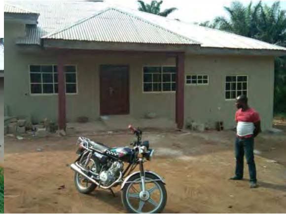
Finished Exterior of the Medical Center
