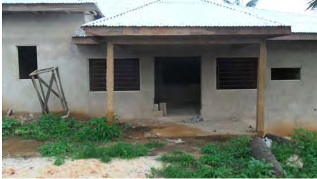
Plastering and Exterior Finishing
