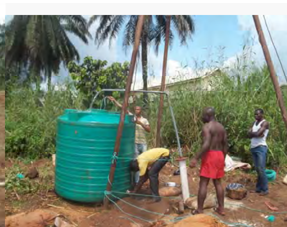
Borehole and Clean Water Installations
